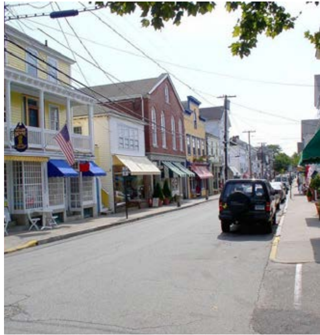
THAMES STREET (facing page, top) has wonderful historic architecture and a sense of intricacy, but rapid traffic and uneven street front development detract from its experience. GROTON RIVERFRONT (facing page, bottom). Revitalization along the water side of Thames Street should take advantage of the double orientation of fronts towards the street and backs opening up onto decks, terraces, and docks on the river.
